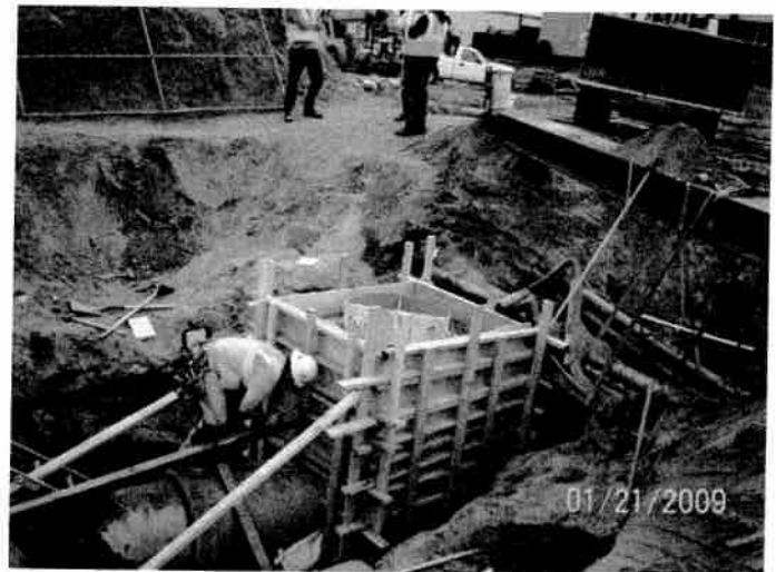
Forming Manhole at Line I
