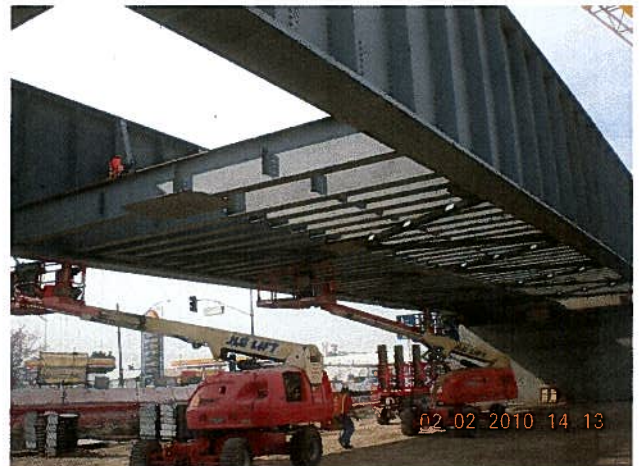
Erecting Sunset Ave Floor Beams
