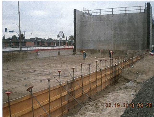
Forming Orange Abutment 2 Footing
