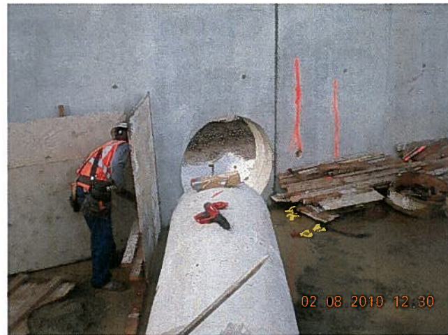
Constructing Drainage Line " Through Main Track RW
