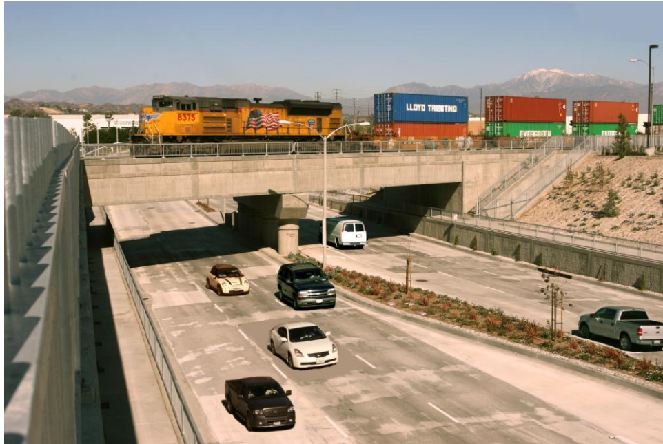
Completed Brea Canyon Road Grade Separation
