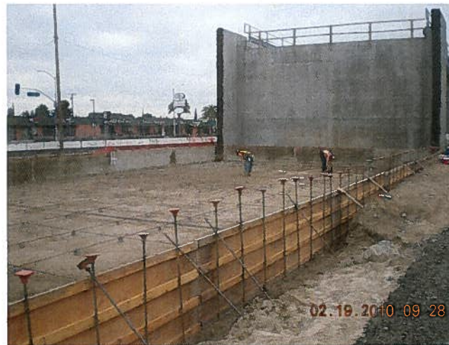
Forming Orange Abutment 2 Footing
