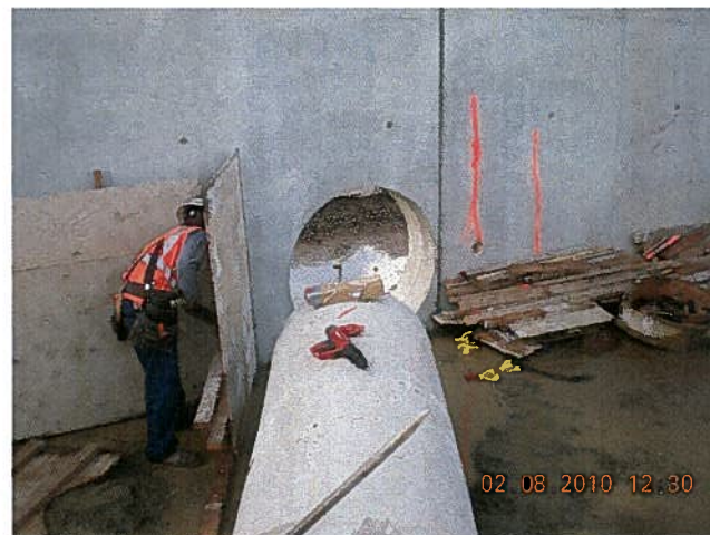
Constructing Drainage Line " Through Main Track RW
