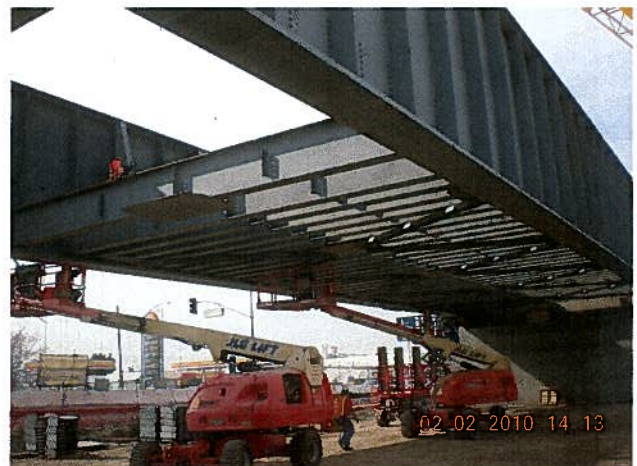
Erecting Sunset Ave Floor Beams
