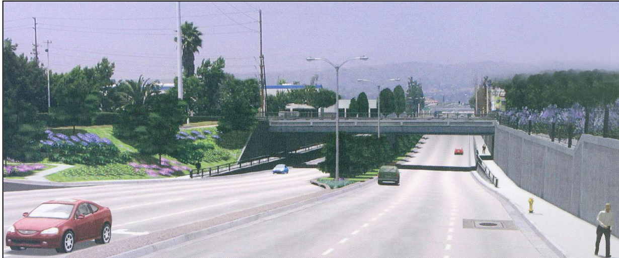
Computer image of the Nogales Street Grade Separation Project. View looking north.
