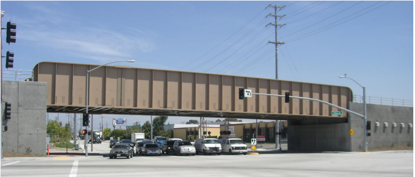
View of completed Sunset Avenue railroad bridge looking north from Valley Boulevard
