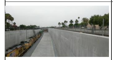
UPRR completed track shift and fully operating on new mainline. Removal of shoofly is complete
