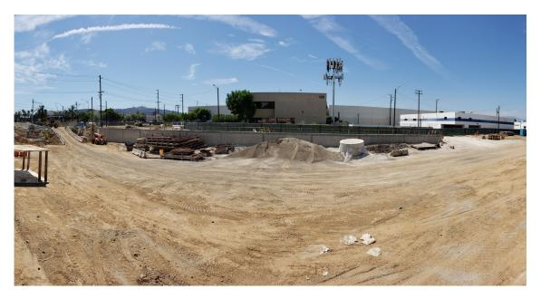
Crews work on excavation and construction of the retaining walls for the roadway underpass north of the railroad tracks. Construction of the Fullerton Road Grade Separation Project includes a four-track railroad bridge, roadway bridge and pedestrian bridge over a six-lane depressed roadway on Fullerton Road, which carries over 23,000 vehicles daily and traversed by 49 trains per day.
