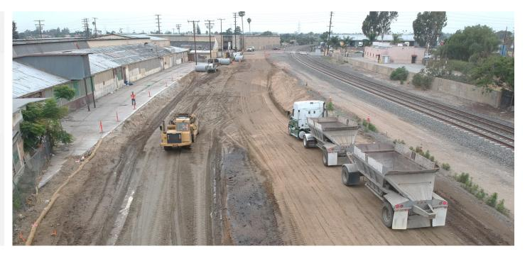
Workers grade the railroad right-of-way to prepare for the installation of a temporary "shoofly" detour track to maintain rail operations during construction of the railroad bridge as part of the Durfee Avenue Grade Separation Project.
