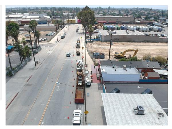
Construction is ramping up with third party utility relocations underway on the Durfee Avenue project site. Crews from various utility companies are relocating gas, electric and fiber optic lines that conflict or run along city streets and the railroad right-of-way prior to construction of the underpass.
