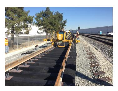
Work is complete on the temporary "shoofly" track constructed to maintain rail operations during construction of the Fairway Drive Grade Separation Project. Upon the successful inspection by Union Pacific Railroad officials, trains will be routed to the shoofly track while crews construct the railroad bridge.
