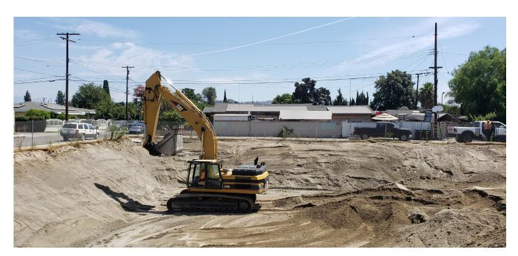
Excavation is underway in advance of construction on the pump station for the Durfee Avenue Grade Separation Project that will remove storm water from the future roadway underpass.
