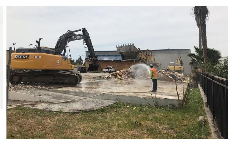
Work started in April on the Durfee Avenue Grade Separation Project in Pico Rivera. Crews have been busy with the demolition of vacant industrial buildings along Durfee Avenue acquired for the project. The grade separation will include construction of a new 1,200-foot-long roadway underpass at the Union Pacific railroad tracks with retaining walls and a 95-foot-long railroad bridge.
