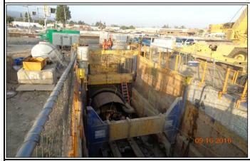
Construction continues on the 78" storm drain. Jacking operation. Verizon completed their relocation within Valley that will allow the contractor to begin structure construction.
