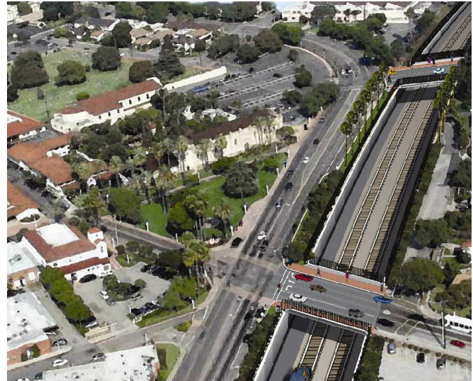
Aerial rendering of the completed trench.
