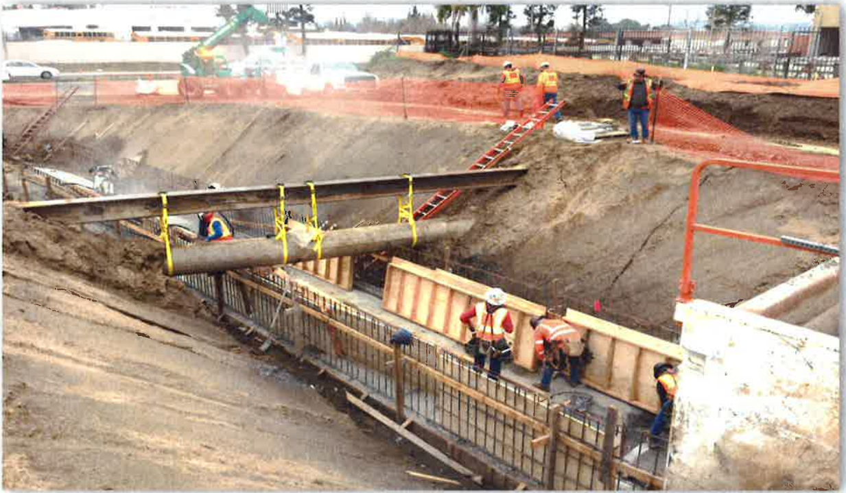
STORM DRAIN INSTALLATION- LEMON AVENUE/60FWY BETTERMENT – CITIES OF DIAMOND BAR & INDUSTRY
