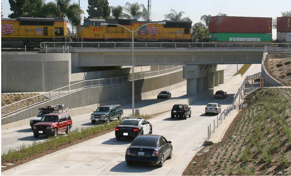
The completed Grade Separation. View looking northeast on Ramona Blvd. toward railroad bridge.
