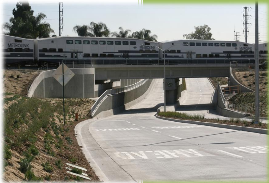
Ramona Blvd. Grade Separation City of El Monte
