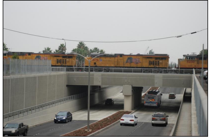
Completed East End Avenue Grade Separation. View looking south on East End Avenue.
