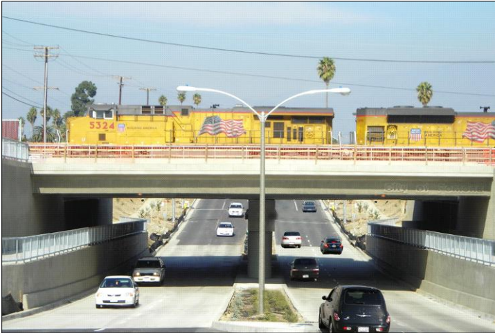
Completed Reservoir Street Grade Separation. View looking north on Reservoir Street.
